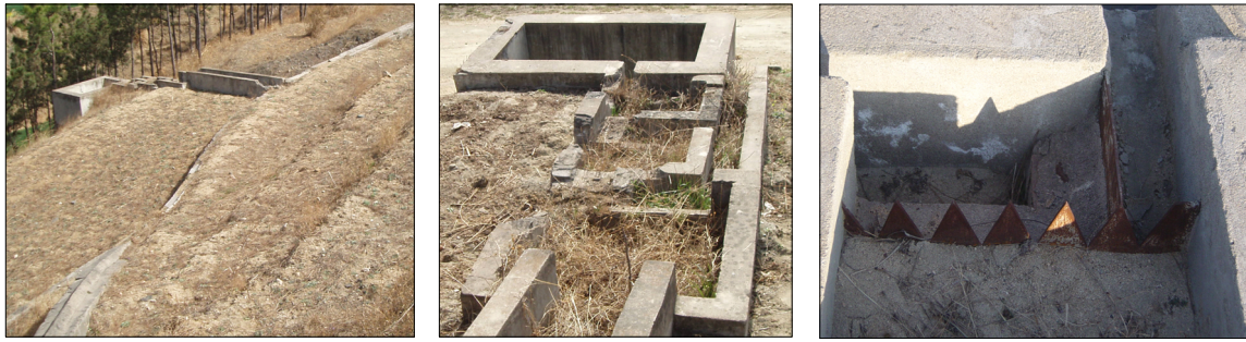
Figure 2. Photos of runoff collection system below an experiment plot (the system shown here was not located at the site described for this study, but is similar to the system that was used).
